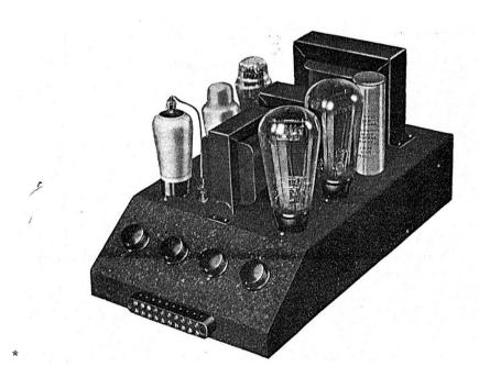
1938. A 12 watt amplifier by Partridge Transformers Ltd, England. Push pull triode output, transformer coupled, no feedback. A very similar 'Quality' unit was also available with an all triode circuit and higher grade transformers. Output transformer integral with the design.
